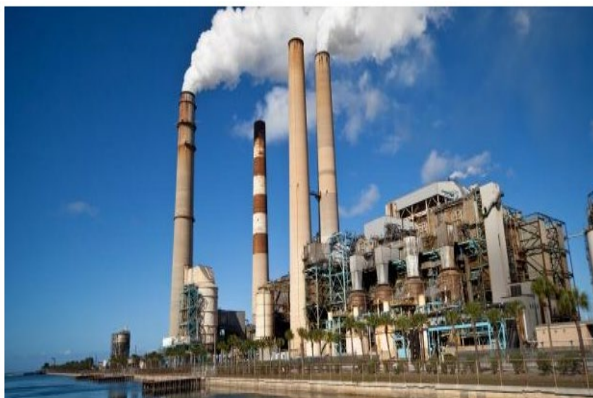
Figure 2. Steam and cogeneration power plants
